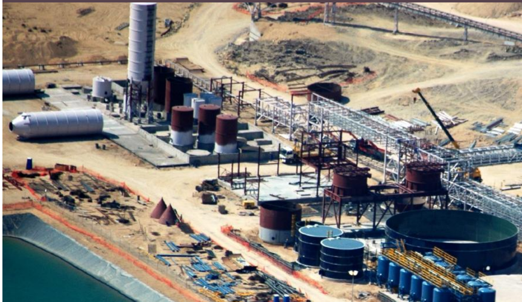
Ion exchange plant at Langer Heinrich Uranium, Namibia
